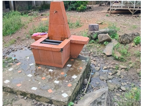
Figure 20: Repair of the water well at Monte Mario
