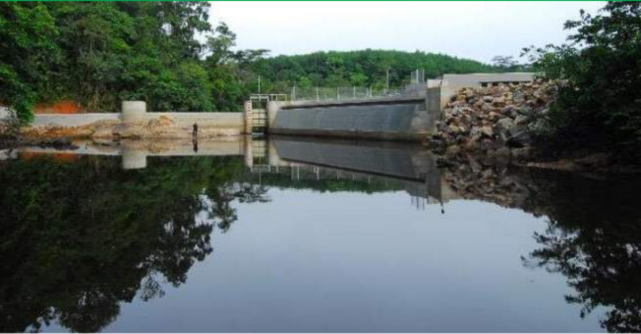
Construction of hydroelectric dam in Liberia (2016)
