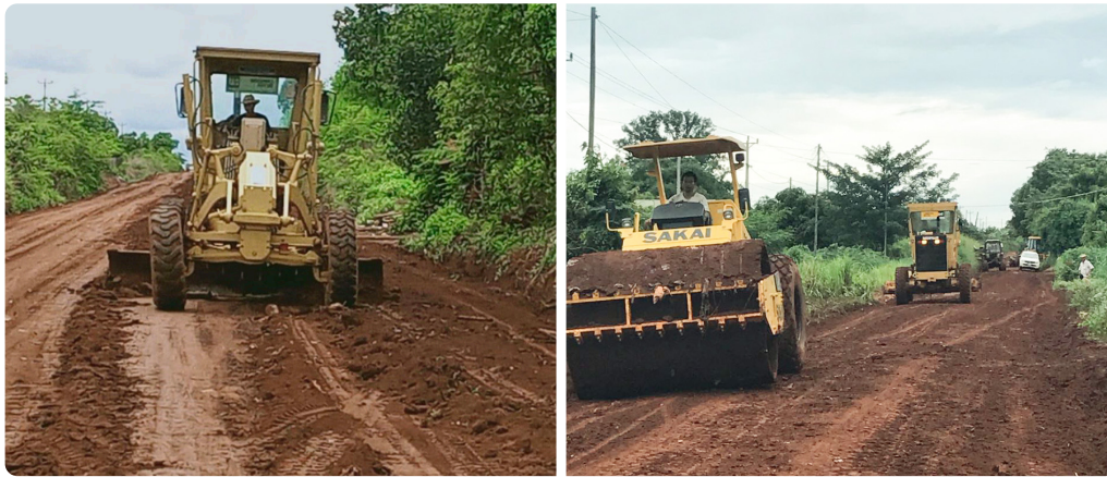
Socfin Cambodia working to fix a road in local village - June 2020
