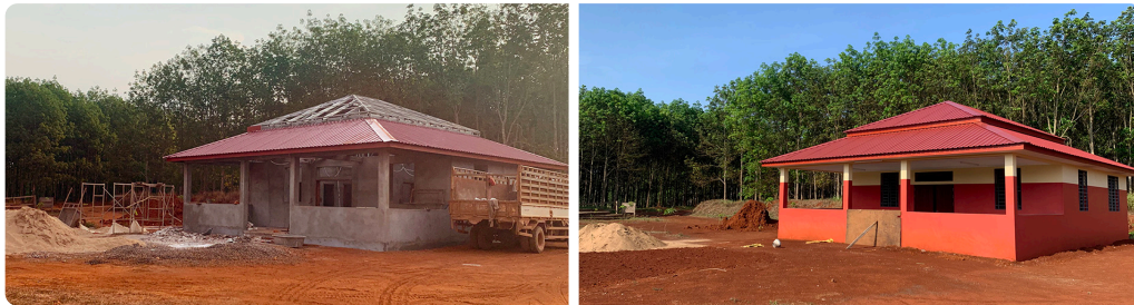
Construction of the new health outpost in Coviphama
