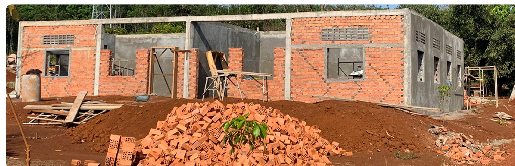
Construction of the new primary school building in Coviphama
