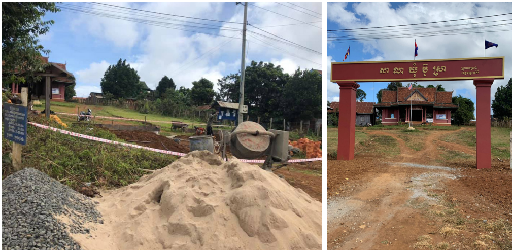
Construction of the public place’s gate – December 2019
