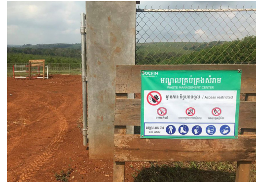
Waste management centre in Coviphama
