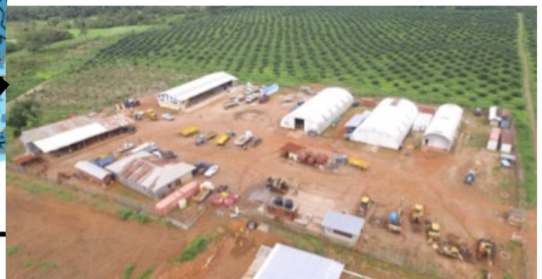
Workshop, garage, fuel Station and storage area
